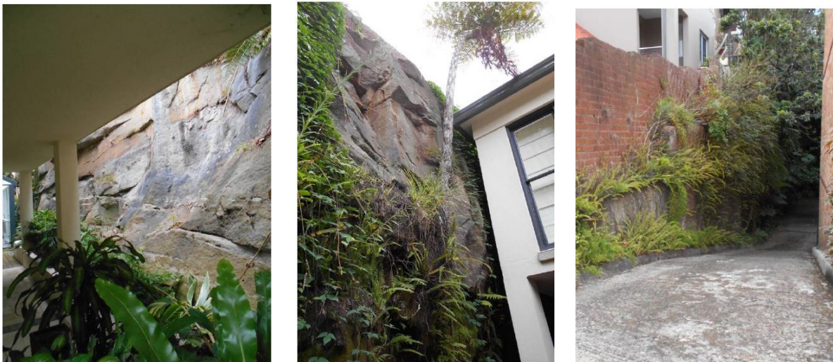
Left and middle: The quarry face to the rear of 65A Avenue Road Right: The quarry rock face along the north of 71 Avenue Road
